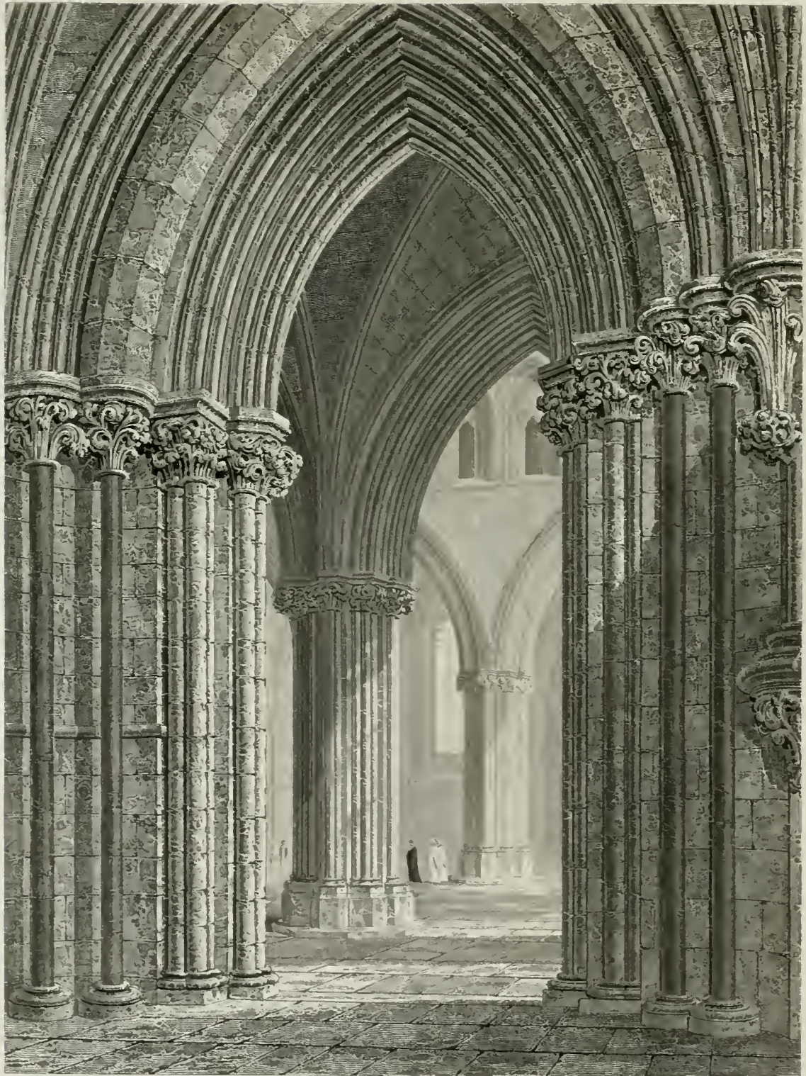
VIEW ACROSS THE NAVE & AISLES
